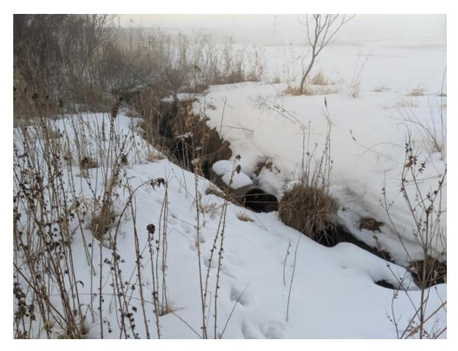
Figure 1: 1922 Main completely exposed and broken above outlet.
